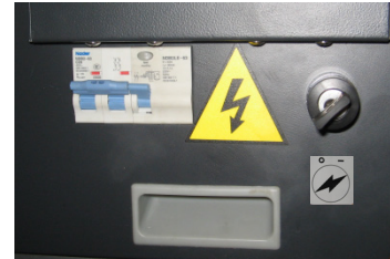
Figure 12. Circuit Breaker (blue bar) On/Off Key
