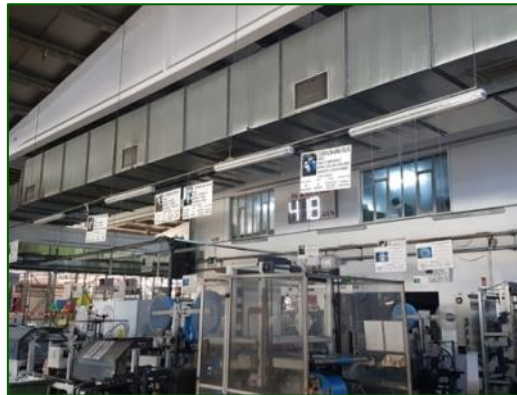
Lighting in production switched off automatically during break times . Outside lighting also controlled automatically
